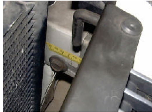
Figure 2 View of the left front bumper attachment bracket at the left frame rail showing 9.5 mm (0.375") of rearward displacement
