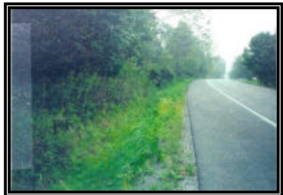
Figure 1. East roadside with drainage ditch
