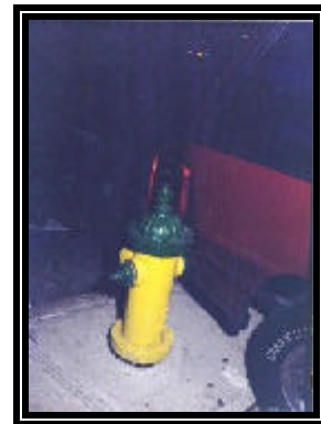
Figure 9. Damage from the fire hydrant
