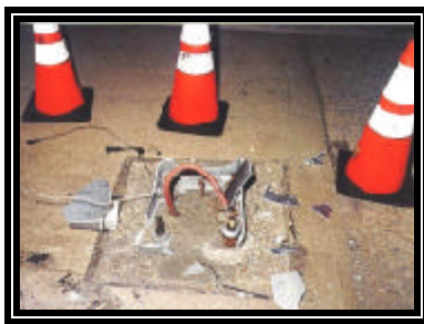
Figure 2. Fractured base of luminaire from the first impact
