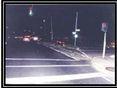
Figure 4. Intersection showing the fractured luminaire in the roadway
