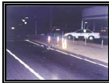
Figure 3. View showing location of the fractured base with respect to the roadway
