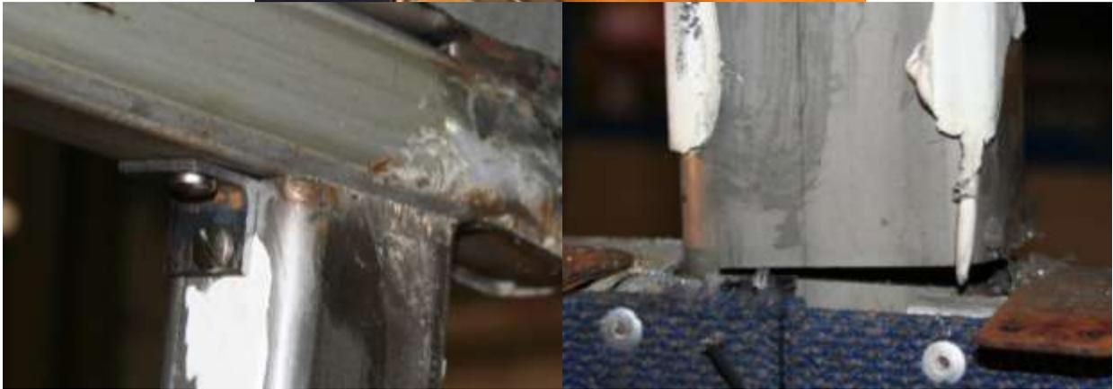
**Figure 3 Window post straightening operation. The top photograph shows the original angle of a bent post. The bottom right photograph shows the notch at the bottom of the post. The bottom left photograph shows the angle bracket with self-tapping screws which reattached the roof to the post.**
