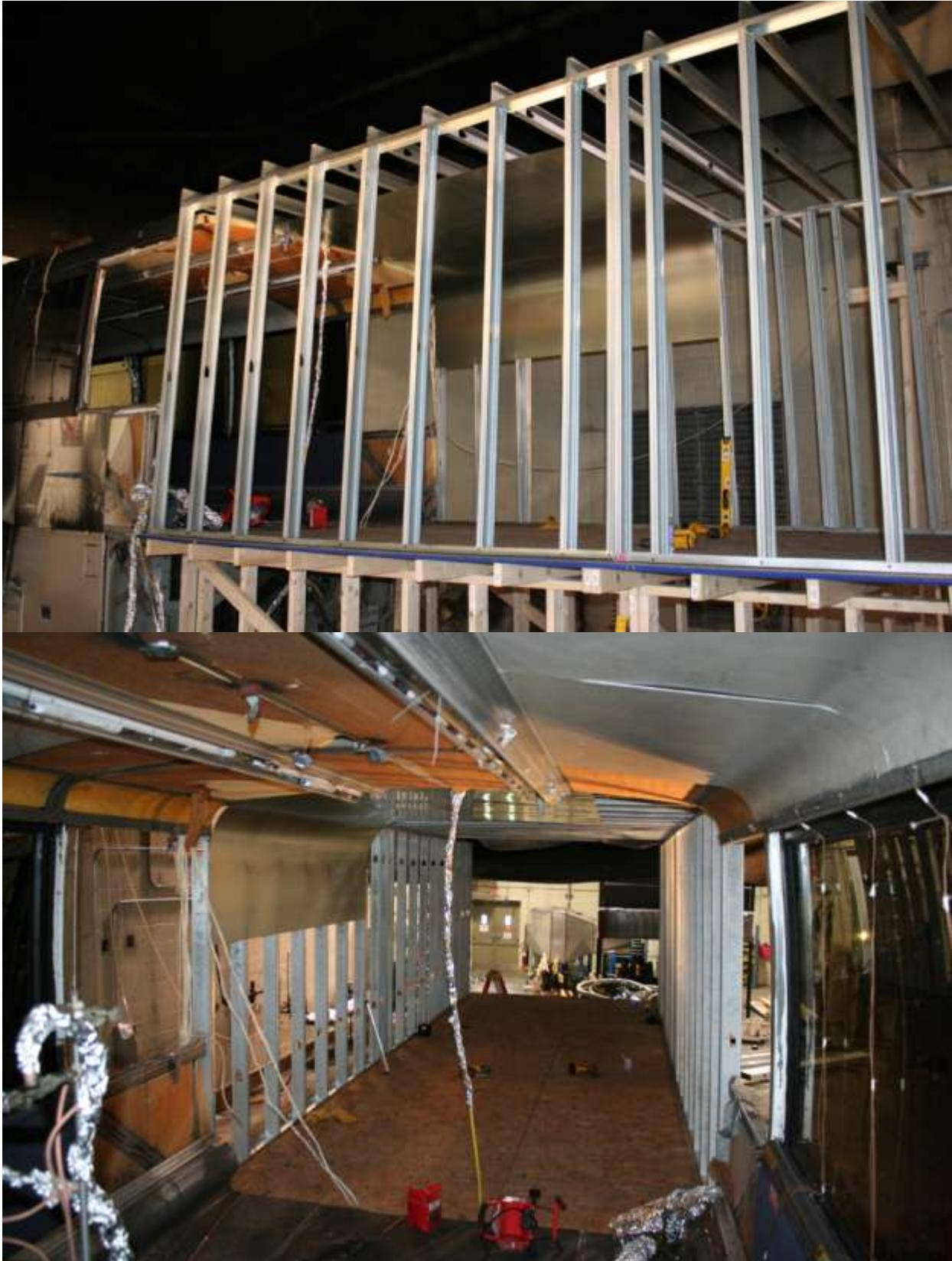
**Figure 12** Two photographs of the motorcoach front extension construction showing the beginning of the attachment of the galvanized sheet steel to the metal studding on the wooden substructure.
