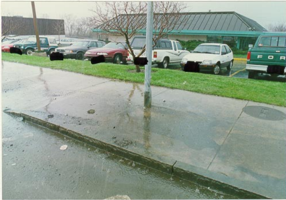
Struck pedestrian signal support pole
