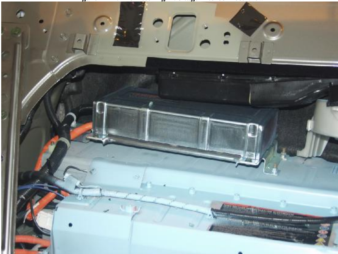
Figure A-12: Post-Test High Voltage Interconnect View
