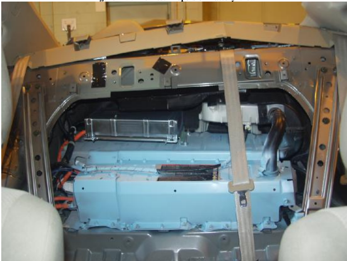
Figure A-10: Post-Test Propulsion Battery View
