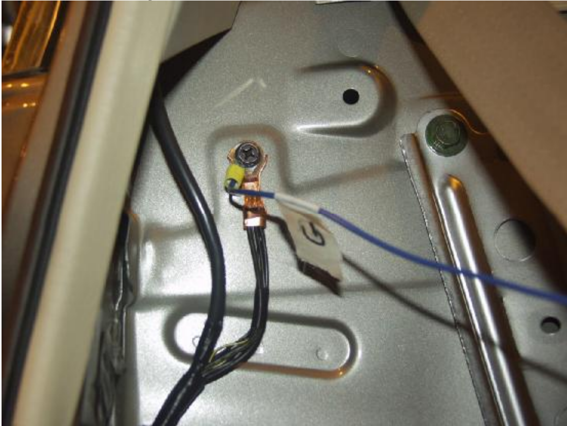
Figure A-6: Pre-Test Chassis Ground Point View
