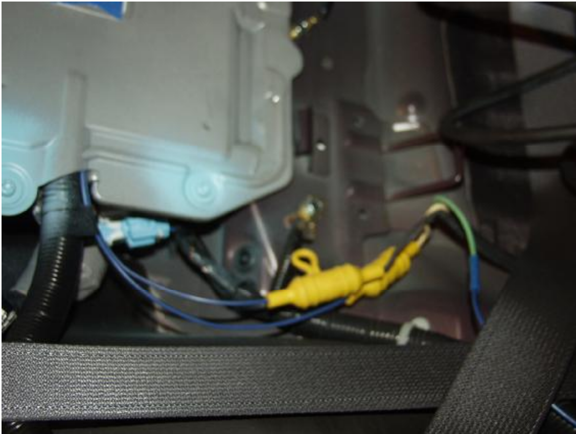
Figure A-11: Pre-Test High Voltage Interconnect View
