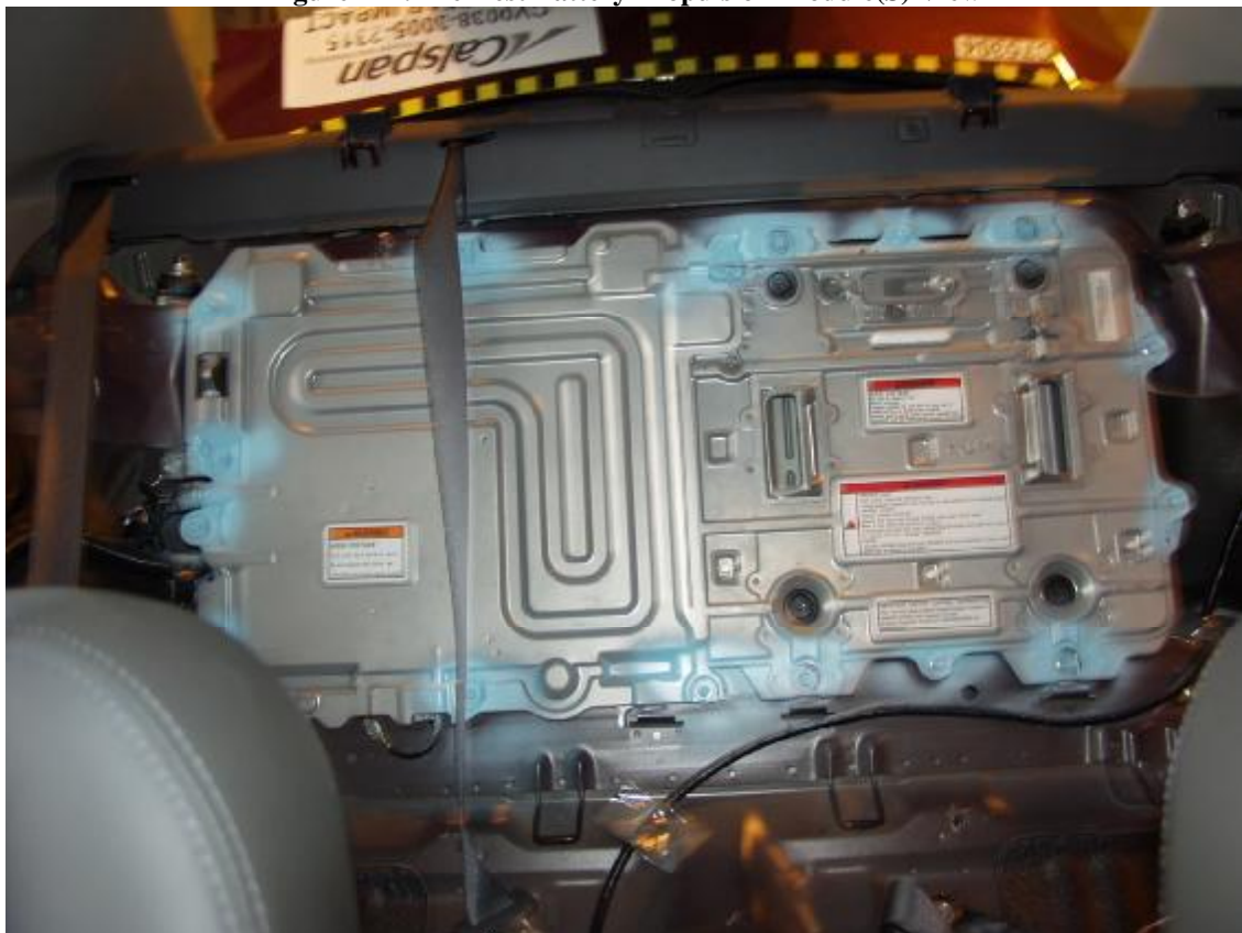
Figure A-8: Post-Test Battery Propulsion Module(S) View
