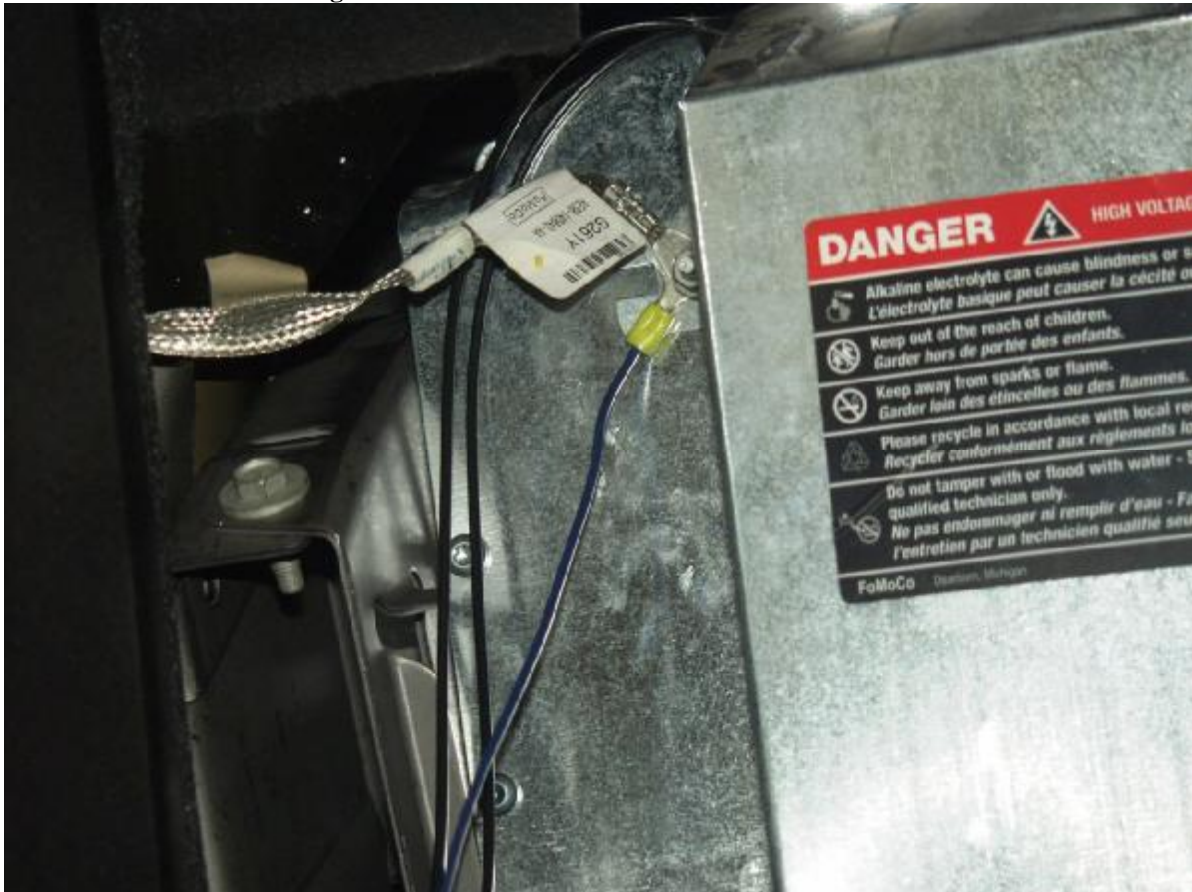
Figure A-6: Pre-Test Chassis Ground Point View
