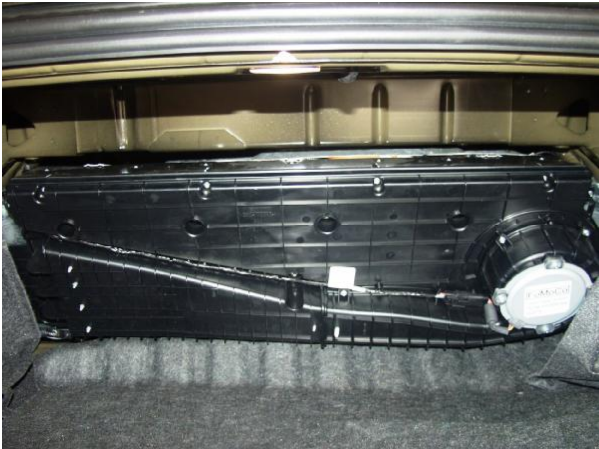
Figure A-41: Pre-Test Battery Venting System View
