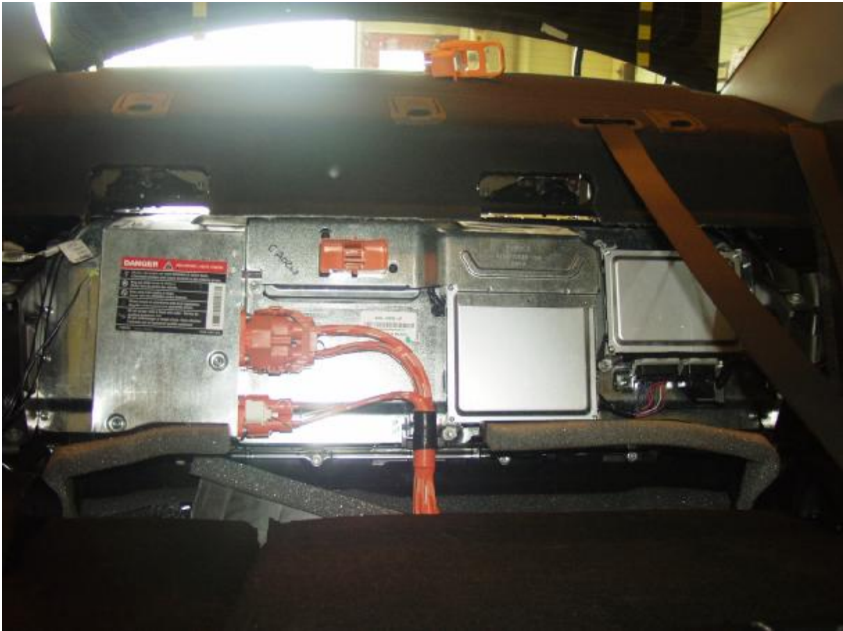
Figure A-33: Pre-Test Battery Propulsion Module(S) View
