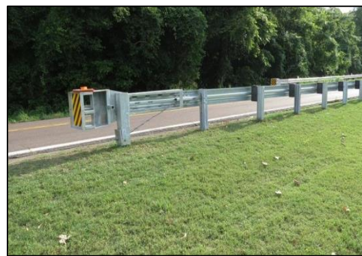
Figure 8: Image depicting an exemplar SKT installation.
