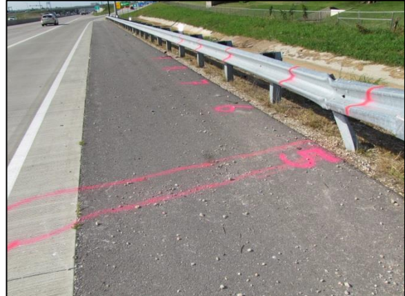
Figure 12: South-looking image from Post 5 of the damaged guardrail.
