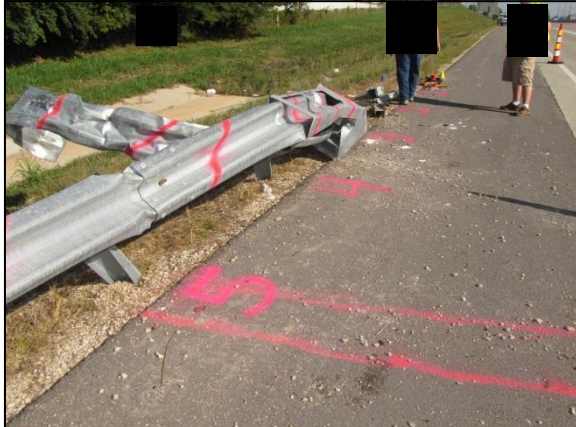
Figure 11: North-looking image from Post 5 of the damaged guardrail.
