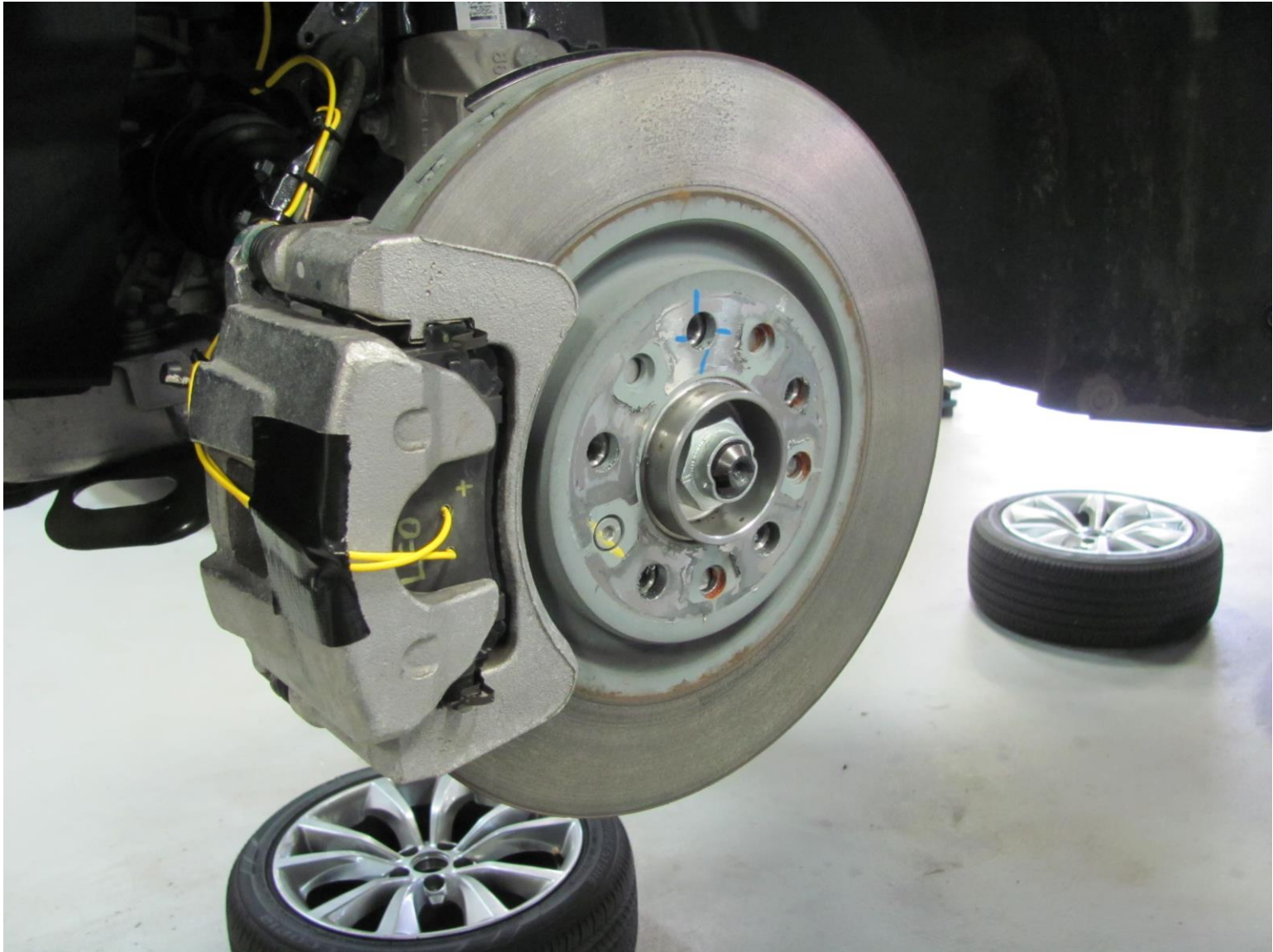
Left Front Thermocouple Installation
