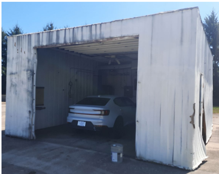
Figure 12. Temporary vehicle storage
