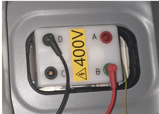
Figure 3. Breakout device installation
