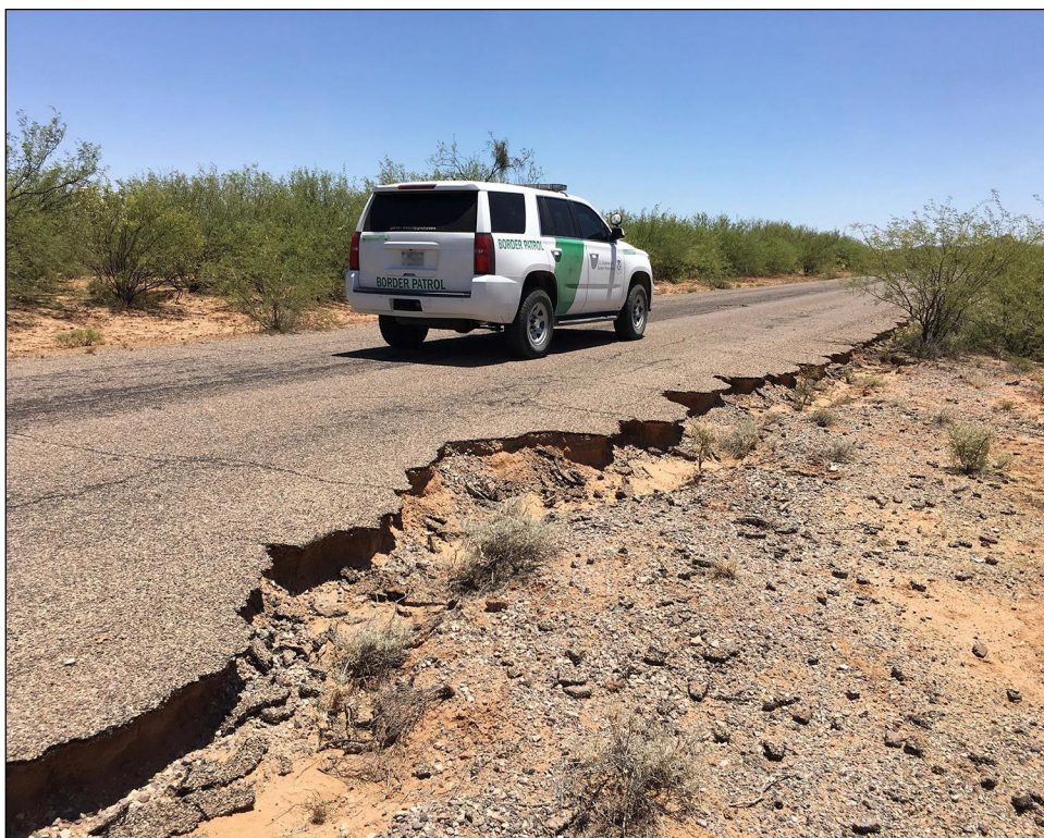
Figure 6: Eroded Conditions on a Tribal Road in Arizona
